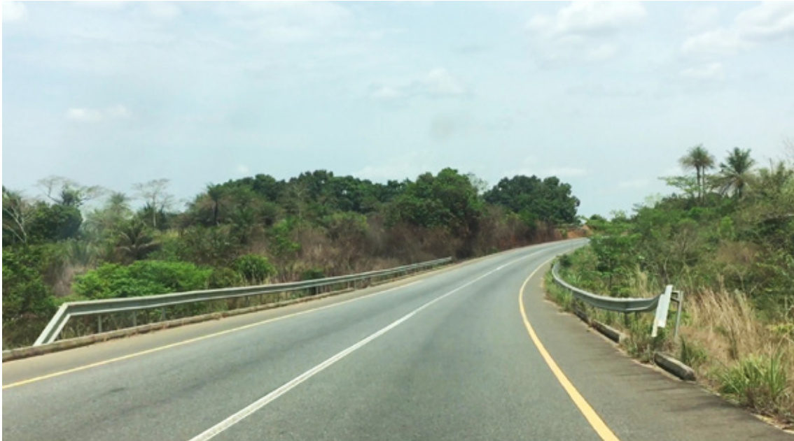
Improved national road network for sustainable development.
